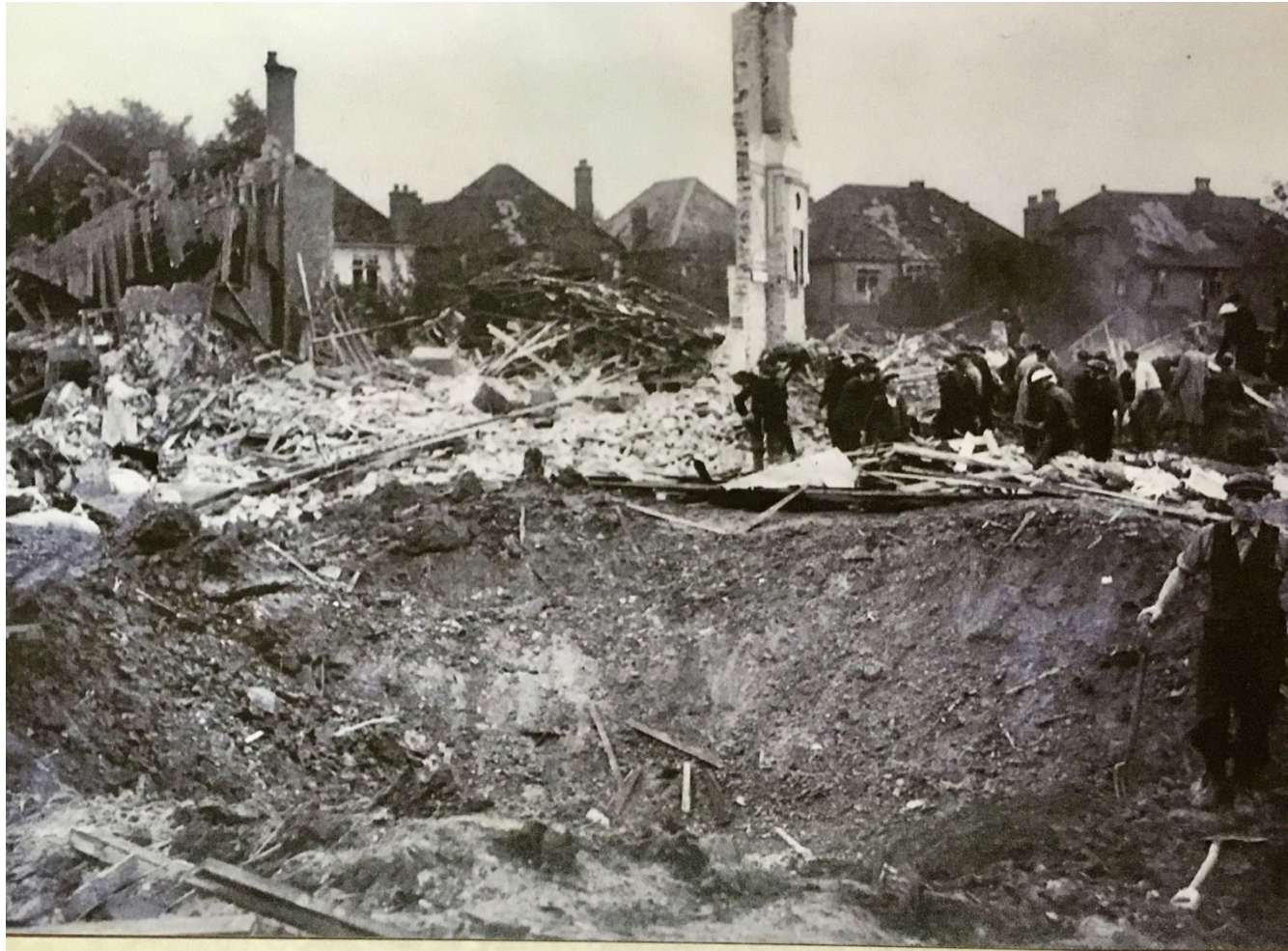
Nos 1 to 5 Staveley Road were almost completely destroyed – the crater is in front of them and you can see the houses of Burlington Lane beyond. The photo was preserved by Special Constable Sydney York, who was sent to "guard the hole"
